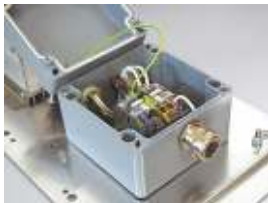
Detailed view of a terminal box
