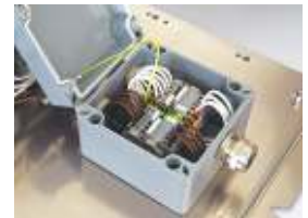
Detailed view of a terminal box
