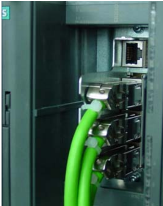
Figure 5-14 Strain relief
